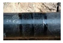
Kebu Bitumen-Tape "Spezial" is a hot-applied corrosion protection tape in accordance with DIN EN 12068 and DIN 30672, load class B at a maximum operating temperature of  $30^{\circ}$ C. The carrier consists of an impregnated synthetic fiber fabric (about  $100 \text{ g/m}^2$ ) and provides high elasticity. Together with the liquid adhesive Kebusol-Primer B III it forms an effective corrosion protection system for steel pipes and fittings.
