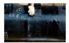
The Kebu Bitumen-Tape GW is a hot applied corrosion protection tape that meets DIN EN 12068 and DIN 30672 and is made of modified bitumen with a high softening and low breaking point. The carrier made of pre-impregnated glass fibre fabric (about  $120 \text{ g/m}^2$ ) makes the tape highly elastic. It meets the requirements of load class B, according to DIN EN 12068, at a continuous operating temperature of up to 30°C.
