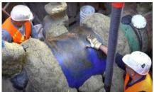
Kebu Priming Paste is a soft brown priming compound based on petrolatum for the preparation of the steel surface prior to the application of Kebu Petrolatum tapes, like Kebu Tape, Kebu Petro Tape A303 or Kebu Tape 90. It is designed to stay elastic and does not dry, crack or harden.
