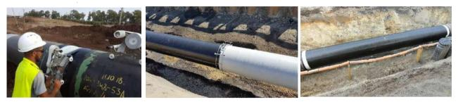
The Kebutyl-System C 50 C is a cold applied two-tape system designed for corrosion protection of pipelines according to DIN EN 12068 (class C 50), DIN 30672 (class C 50) and ISO 21809-3 type 12A-1 ( $T_{max}$  50°C).
