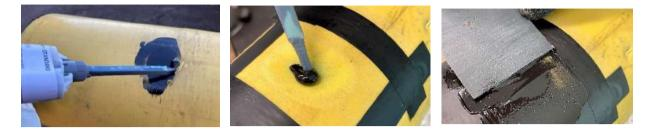
Kebudur PU Repair is a two-component polyurethane for repairing of defects and mechanical damages on PE- and PP-factory coating. It is also used for the coating of fittings and pipes.
