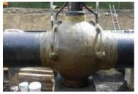
Kebu Petro Tape A303 is a cold applied corrosion protection tape. It consists of modified petroleum products, a synthetic fiber fabric as an insert and a laminated PE film. The Kebu Petro Tape A303 meets the requirements of DIN EN 12068 and DIN 30672, load class A, maximum continuous operating temperature up to 30°C.
